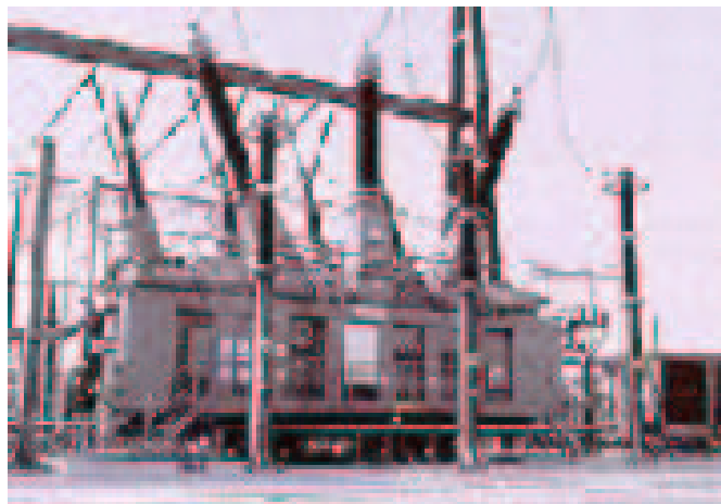
Figure 2.2. A 500 MVA Power Transformer. (Courtesy of ABB)
