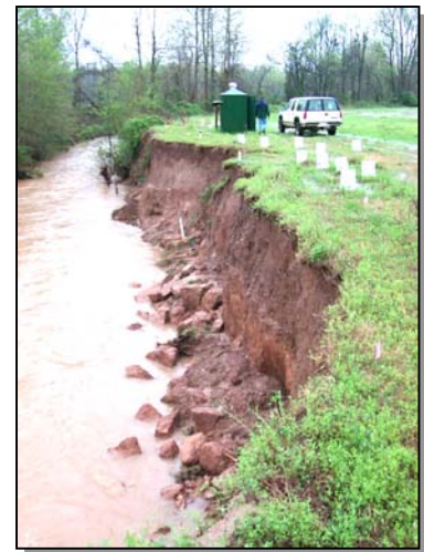
Stream bank stability research in NSL experimental watersheds
